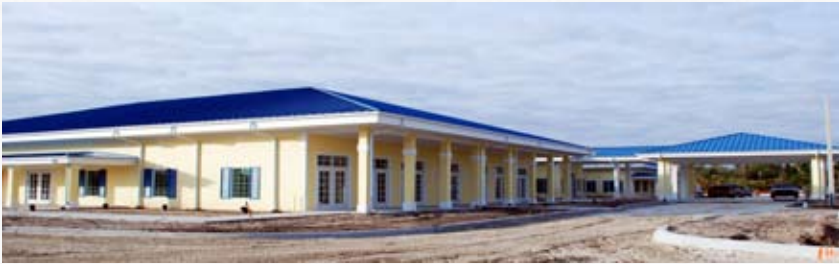
During 2010, The Council on Aging celebrated the expansion of their organization into this new 34,256 Sq. Ft. commercial building in Stuart, financed by Gulfstream Business Bank.
